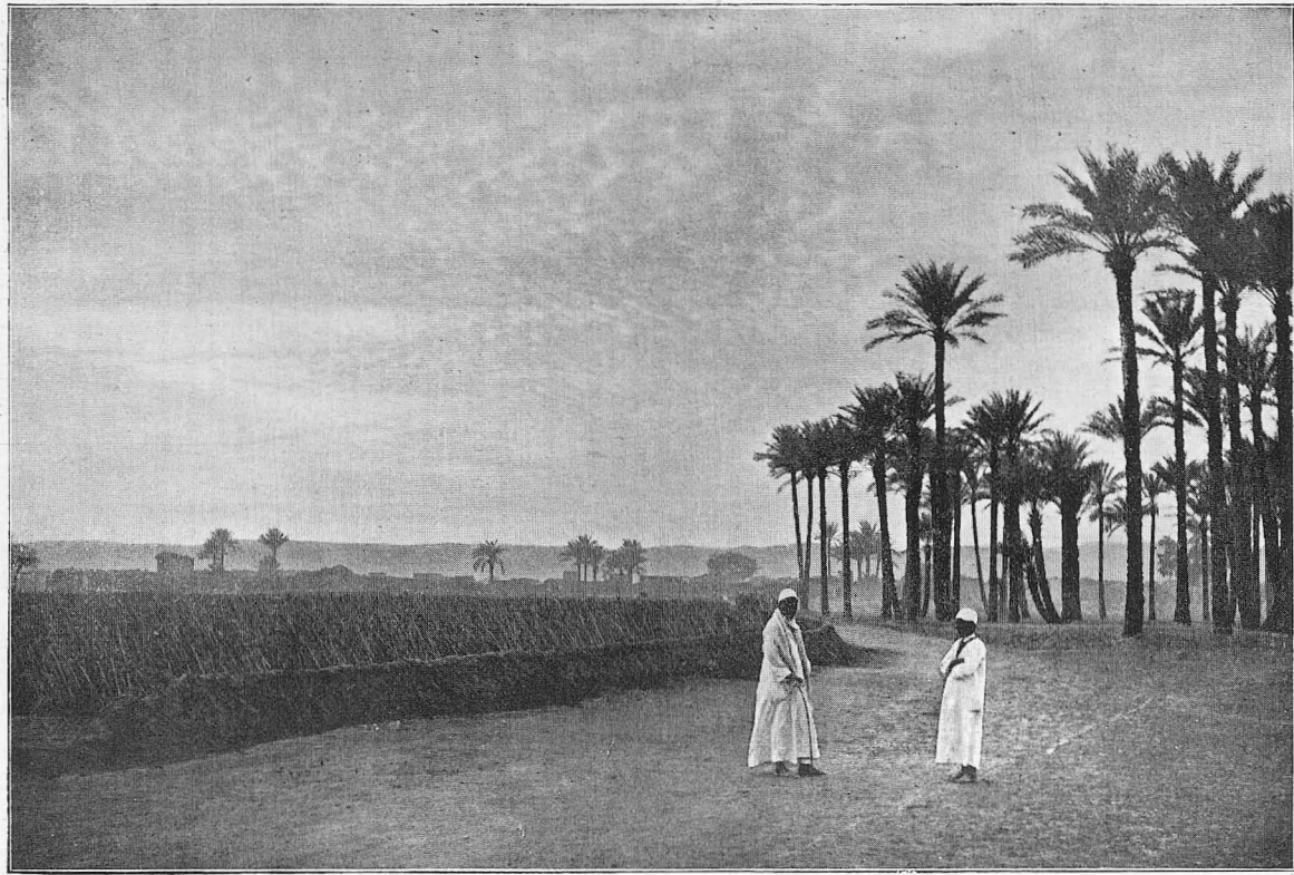
A CANAL EMBANKMENT.
